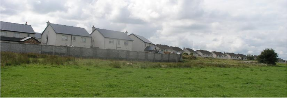
Figure 13.9: Southern block wall boundary
